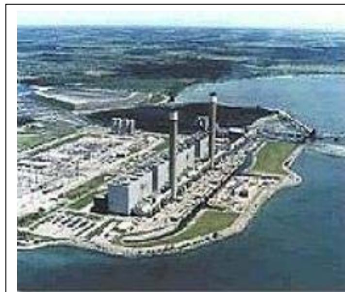
Ontario Power Generation's coal-fired thermal generating station in Nanticoke, Ontario
