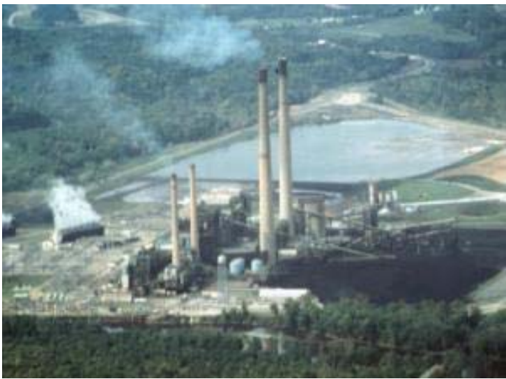
Coal-fired power plant in Ohio << photo courtesy of Ohio EPA >>
